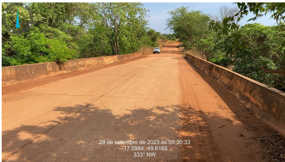
Km: 5,70 – Ponte de Concreto Armado 40 x 8,40.
