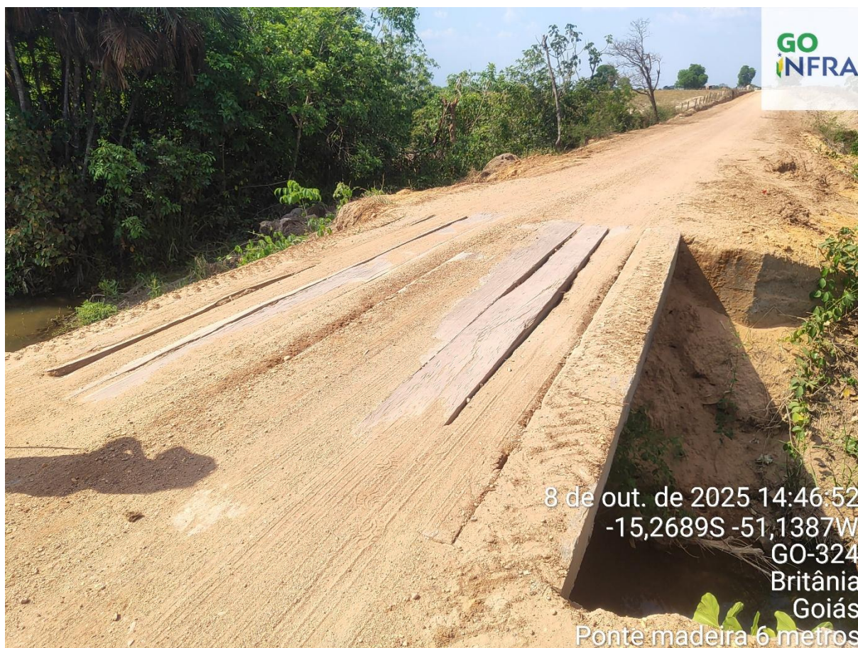
Km 45,3 – Ponte de madeira 6,0 m
