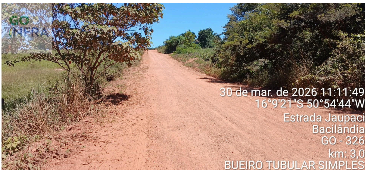
Km 3,0 — Bueiro Tubular Simples
