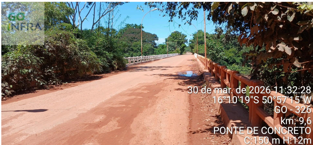
Km 9,6— Ponte de Concreto C:150m H:12,0m
