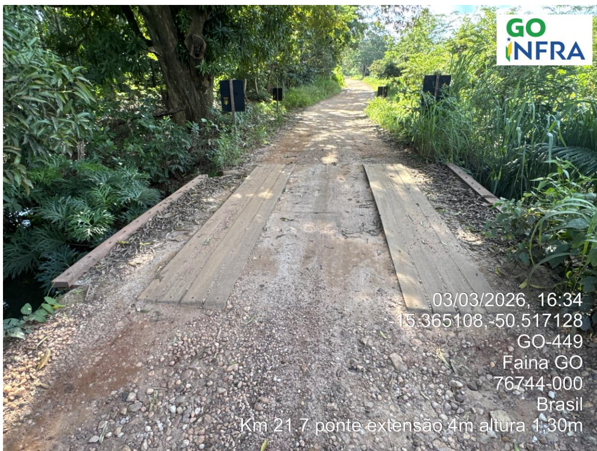
Km 21,7 – Ponte de Madeira C: 4,0m H:1,3m
