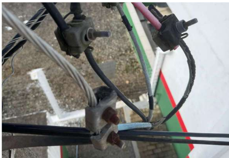
Figura 9-Conector neutro inadequado
