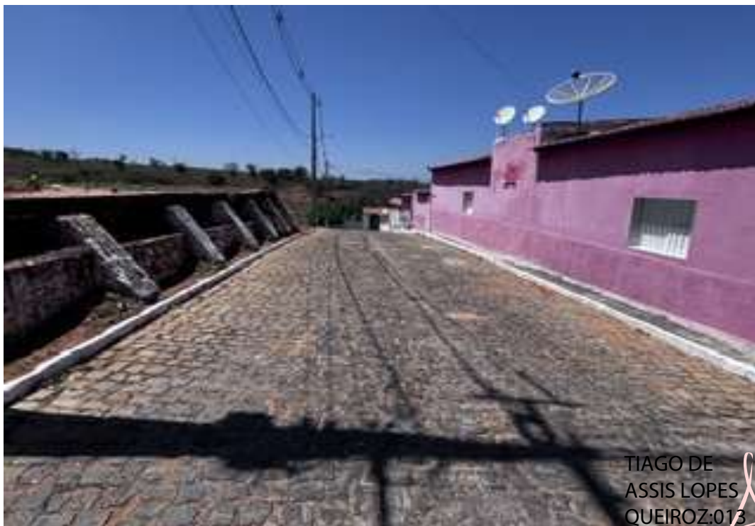
TRAVESSA MANOEL JOSÉ DE BESSA
