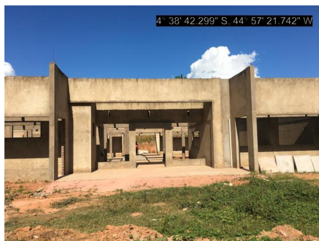
FOTO 6 - VISTA FRONTAL PRINCIPAL – 26/06/2024
