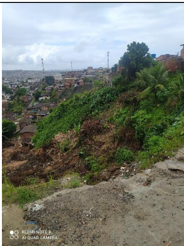
Figura 11: VALE NO TALUDE
