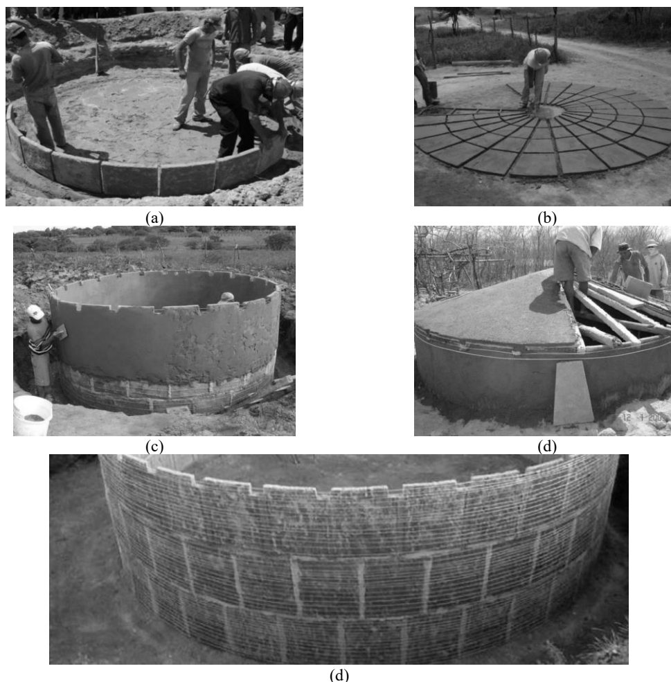
Figure 1 - a) Positioning of the first row of plates; (b) Casting of the plates; (c) Coating of the walls; (d) Execution of the walls; (e) Detail of the arrangement of steel wires (ASA [6])
