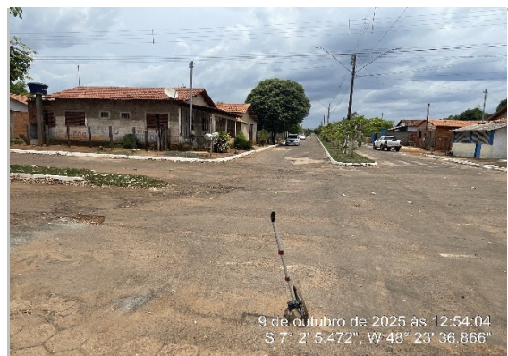
RUA RECAPEAMENTO CBUQ -7.034819, -48.393556
