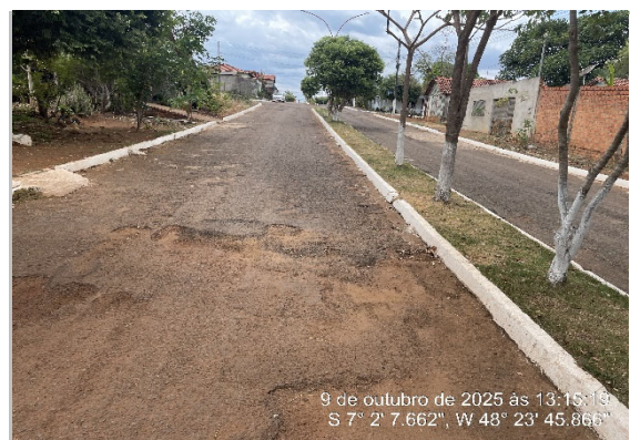
RUA RECAPEAMENTO CBUQ -7.035275, -48.396153
