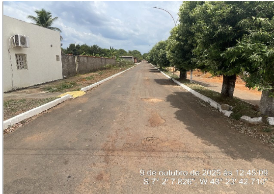
RUA RECAPEAMENTO CBUQ -7.035347, -48.395128
