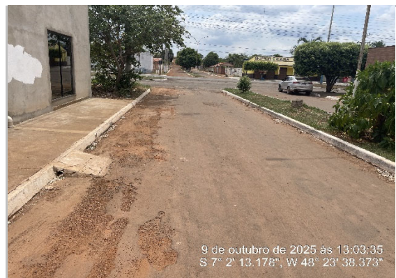
RUA RECAPEAMENTO CBUQ -7.037056, -48.394239
