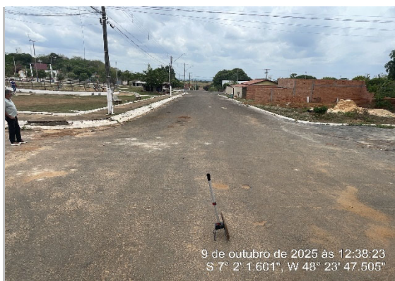
RUA RECAPEAMENTO CBUQ -7.033758, -48.396636
