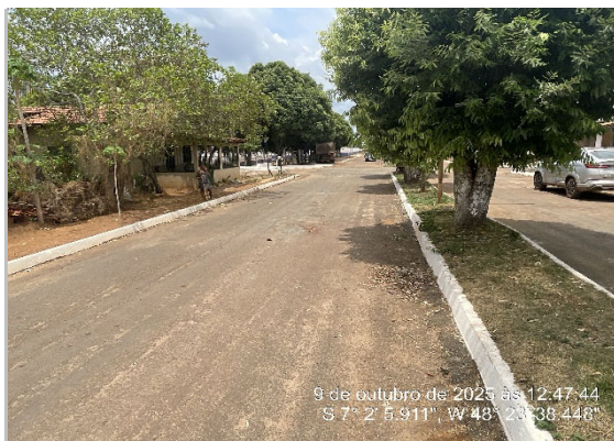
RUA RECAPEAMENTO CBUQ -7.034911, -48.393825
