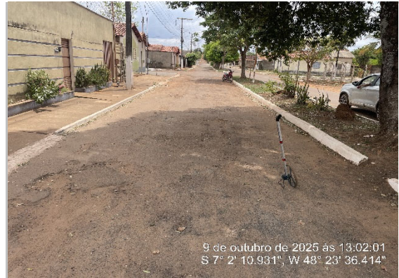
RUA RECAPEAMENTO CBUQ -7.036747, -48.393353
