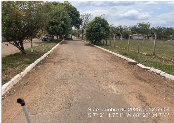
RUA RECAPEAMENTO CBUQ -7.036642, -48.393089
