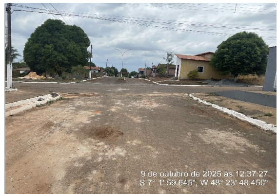
RUA RECAPEAMENTO CBUQ -7.03365, -48.396664
