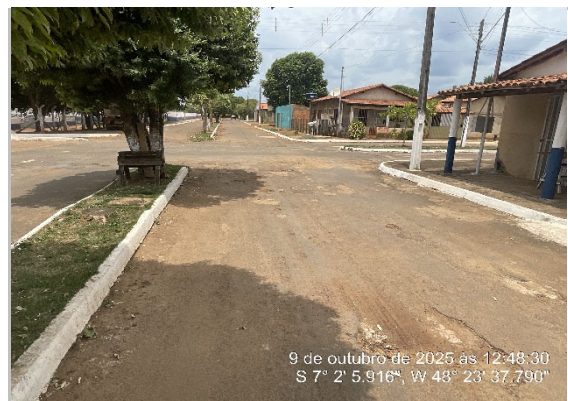
RUA RECAPEAMENTO CBUQ -7.034983, -48.393703
