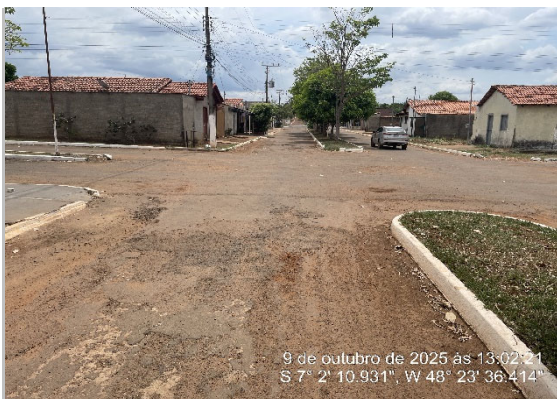
RUA RECAPEAMENTO CBUQ -7.036808, -48.393553
