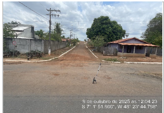
RUA RECAPEAMENTO CBUQ -7.031253, -48.396533
