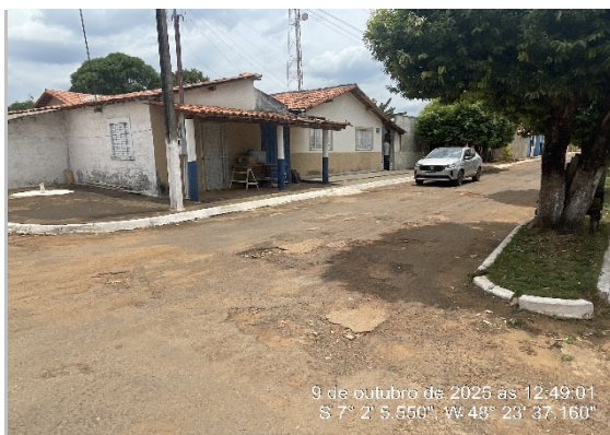
RUA RECAPEAMENTO CBUQ -7.03485, -48.393586
