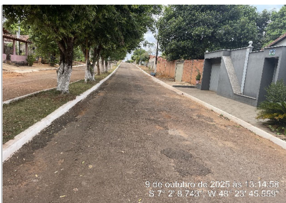
RUA RECAPEAMENTO CBUQ -7.035436, -48.396078
