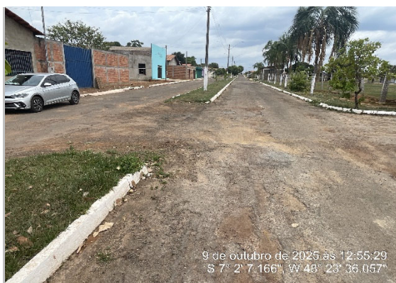
RUA RECAPEAMENTO CBUQ -7.035356, -48.393383
