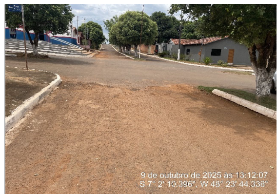
RUA RECAPEAMENTO CBUQ -7.035869, -48.396175
