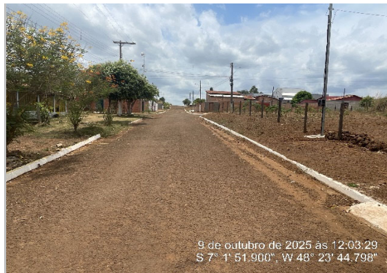
RUA RECAPEAMENTO CBUQ -7.031111, -48.396014
