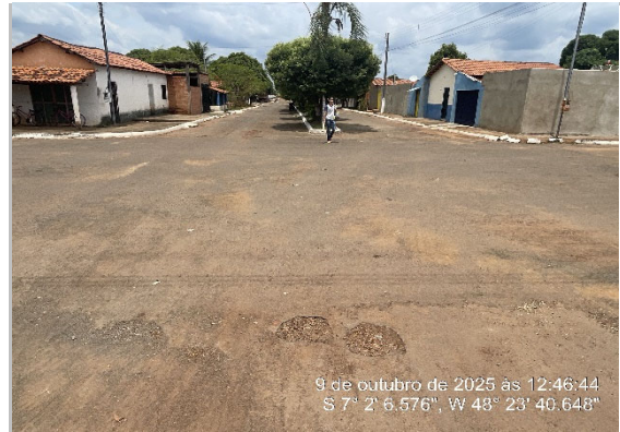
RUA RECAPEAMENTO CBUQ -7.035108, -48.394356
