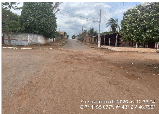
RUA RECAPEAMENTO CBUQ -7.033019, -48.396739
