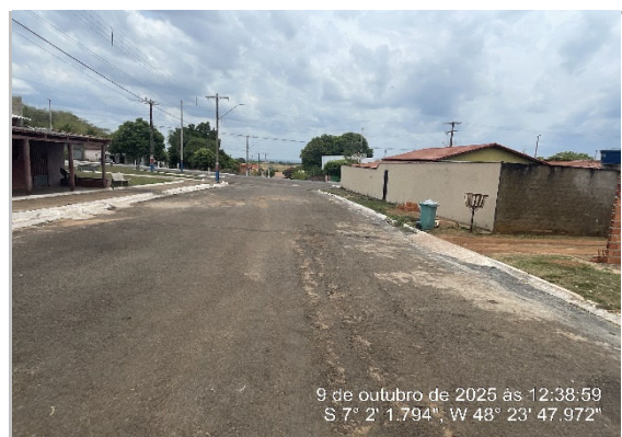
RUA RECAPEAMENTO CBUQ -7.033719, -48.396356
