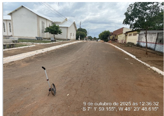
RUA RECAPEAMENTO CBUQ -7.033056, -48.396861
