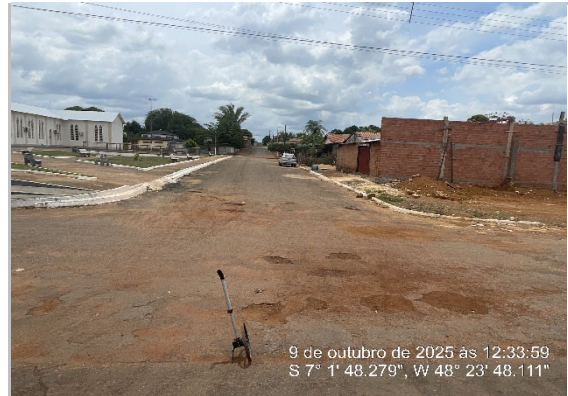
RUA RECAPEAMENTO CBUQ -7.032778, -48.396014
