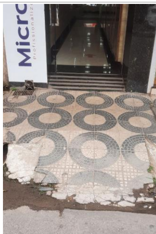
Rampas de acesso as salas
