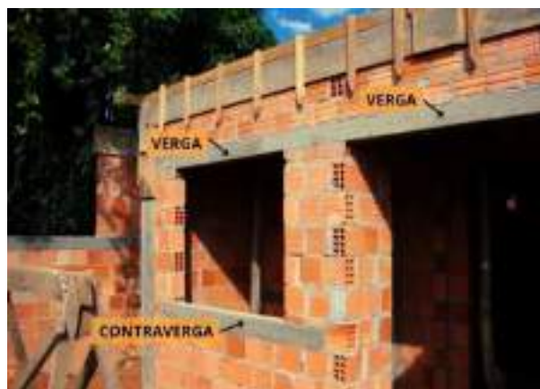
Figura 15 – Verga e Contraverga moldada in Loco
