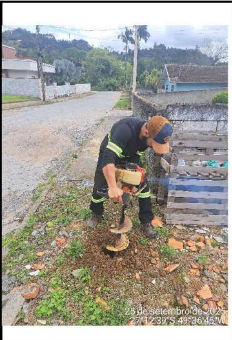
CBR-35 Rua João Cavilla
